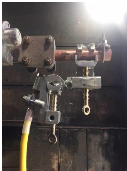
Photo 5: Double Energized Setup
